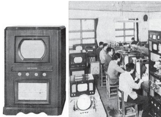
Prototype of a console-model TV with a 12-inch CRT (cathode ray tube) (1951) (left)
